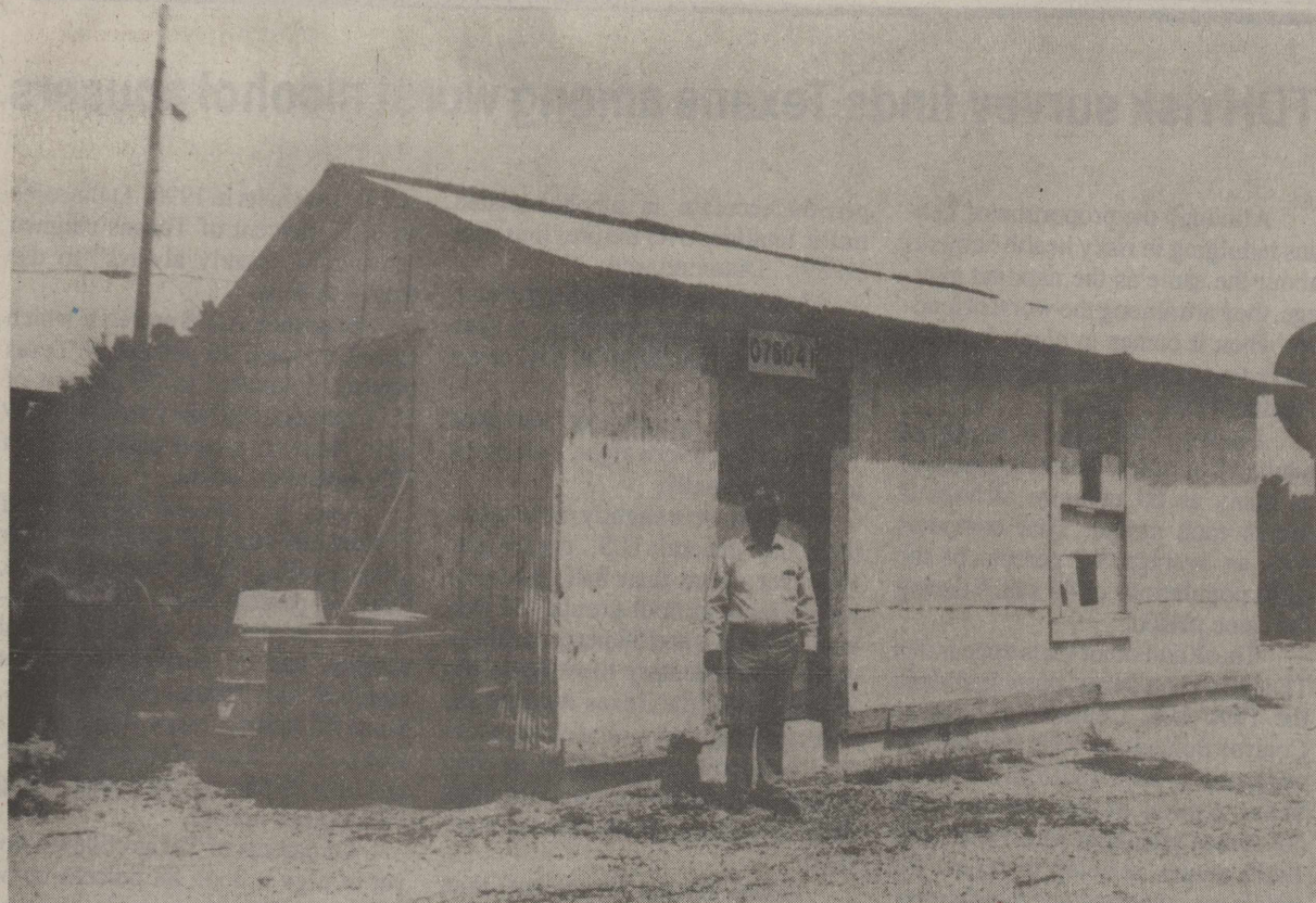
ROSALIO LONGORIA STANDS BEFORE THE ORIGINAL STATE HIGHWAY DEPARTMENT OFFICE which was in use when he began working there 31 1/2 years ago. The building was moved from south of the interstate to the department's new location and is used for storage.
