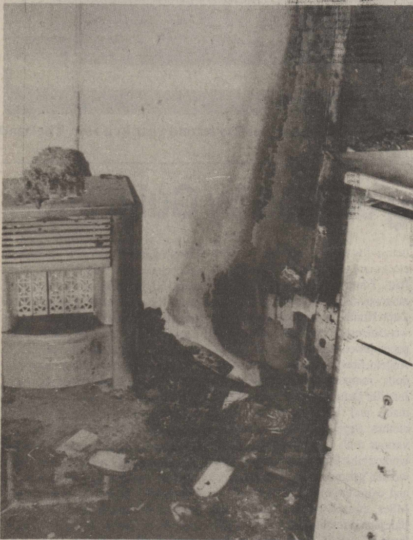
The Lucas Longoria home at 525 Heraclio St. received damage to a bedroom when a fire started from a space heater on Sunday.
