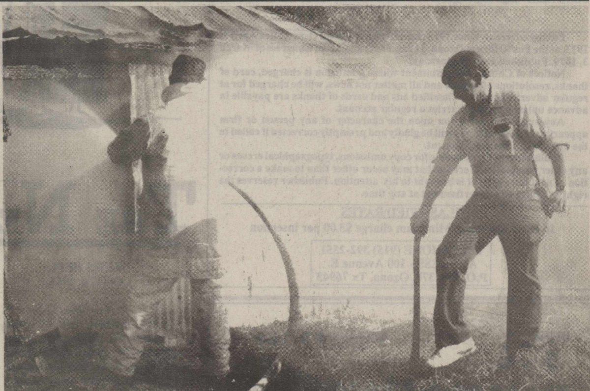
Heavy damage resulted from a garage fire October 2 at 508 Ave. J. Children playing with matches are believed to be the cause of the blaze according to arson investigator Steve Kenley. The building was totally involved when firemen arrived after receiving the 4:46 p.m. call. Naomi and Eddie Galindo are residents at the property.
