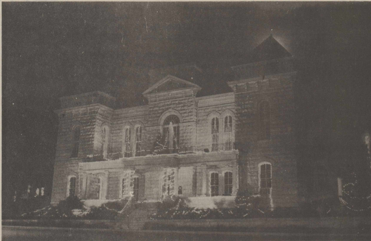
The Crockett County Courthouse tied for first place the public building division of the decorating contest.
