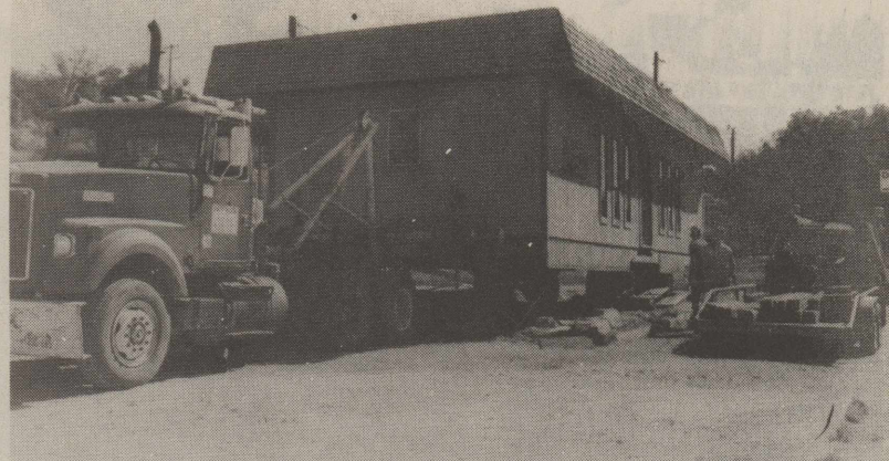
The Donut Shop building is pictured being prepared to be moved. Tina and David Wells have purchased the building and will open a donut shop in McCamey. Tina is the sister of Jan Lott.
