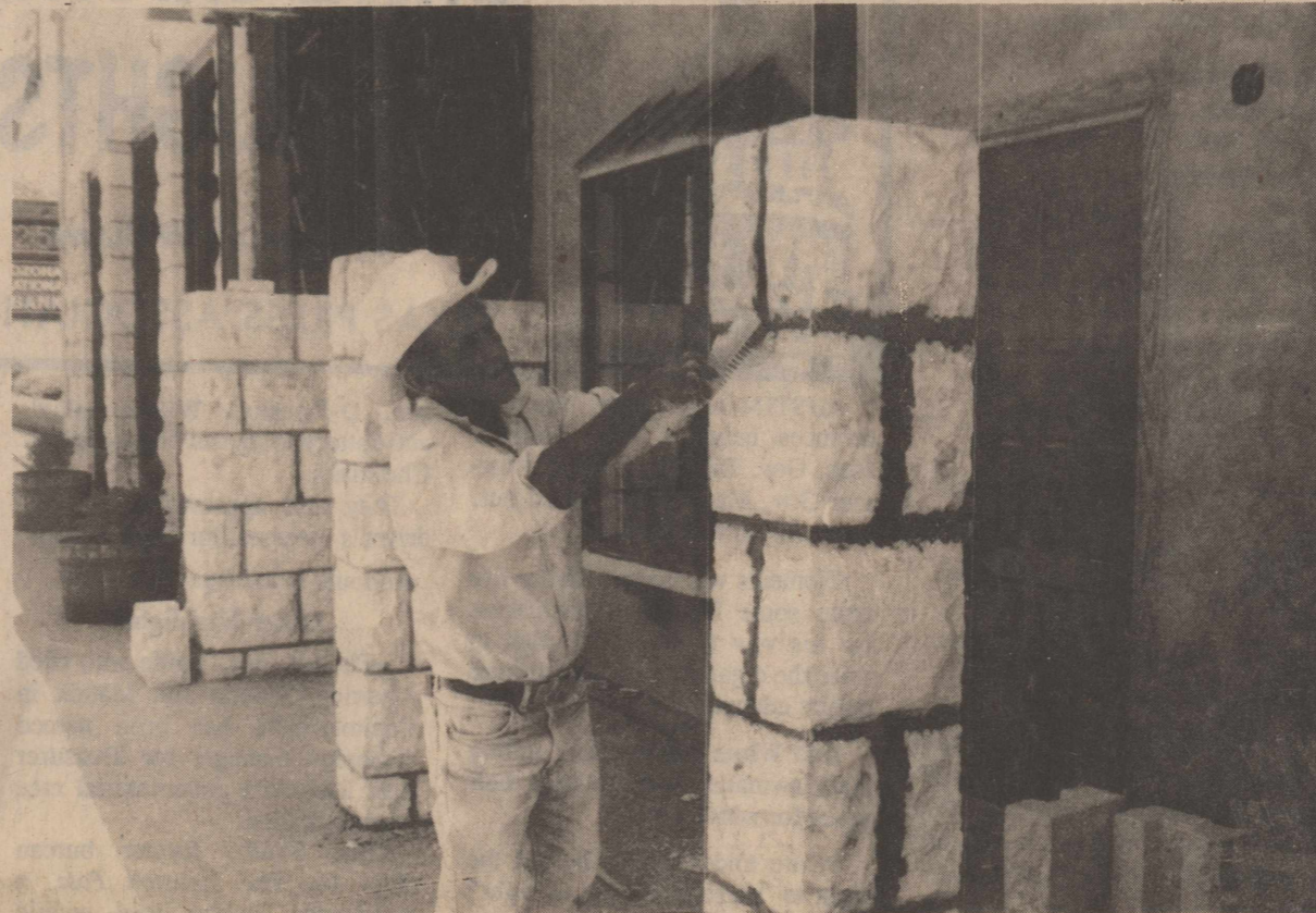
Moses Coy removes excess mortar from limestone blocks he is placing as supports at The Crockett
