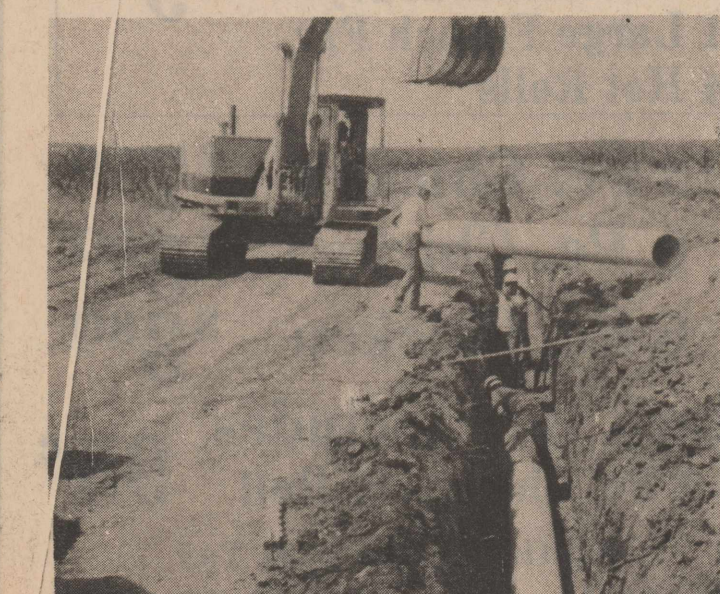
Laying pipeline to the treatment plant.
