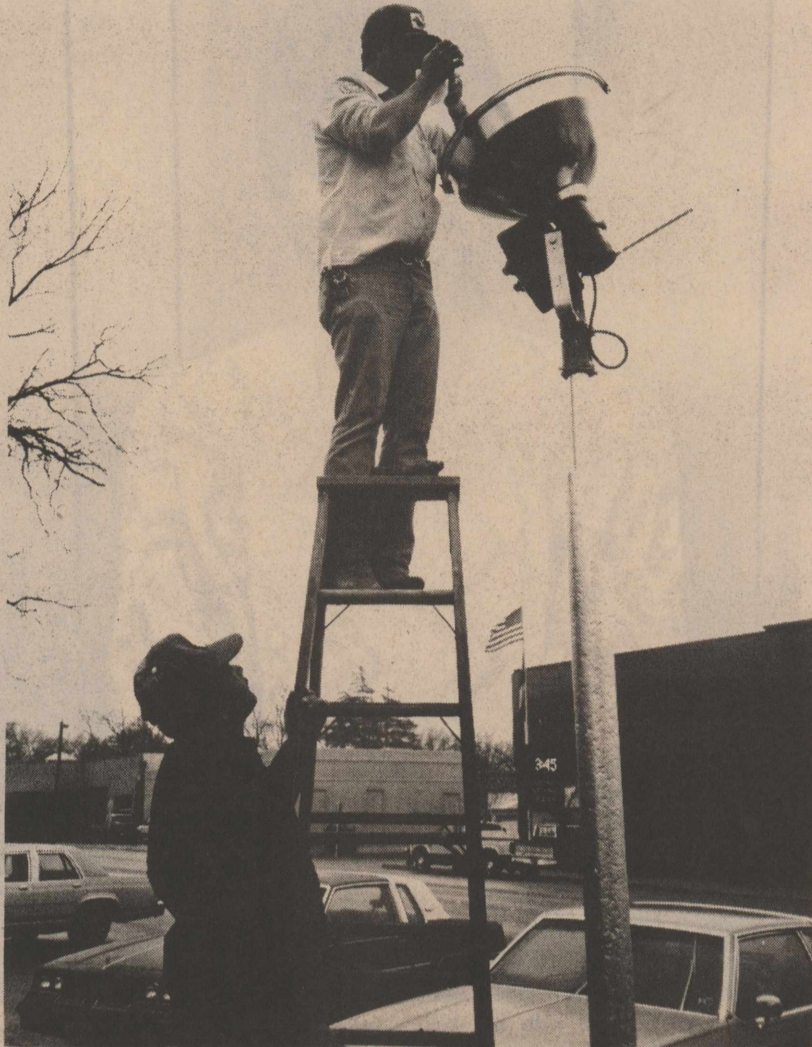
A HIGH DENSITY LIGHT was installed last week to come on at sundown and click off at sunup. Focused on the all-weather flag and the Davy Crockett statue, the flags will stay up day and night. Drilling holes in the frame to allow water to escape is Doug Meador of the Water District and assisted by Charlie Ramos, employee.
