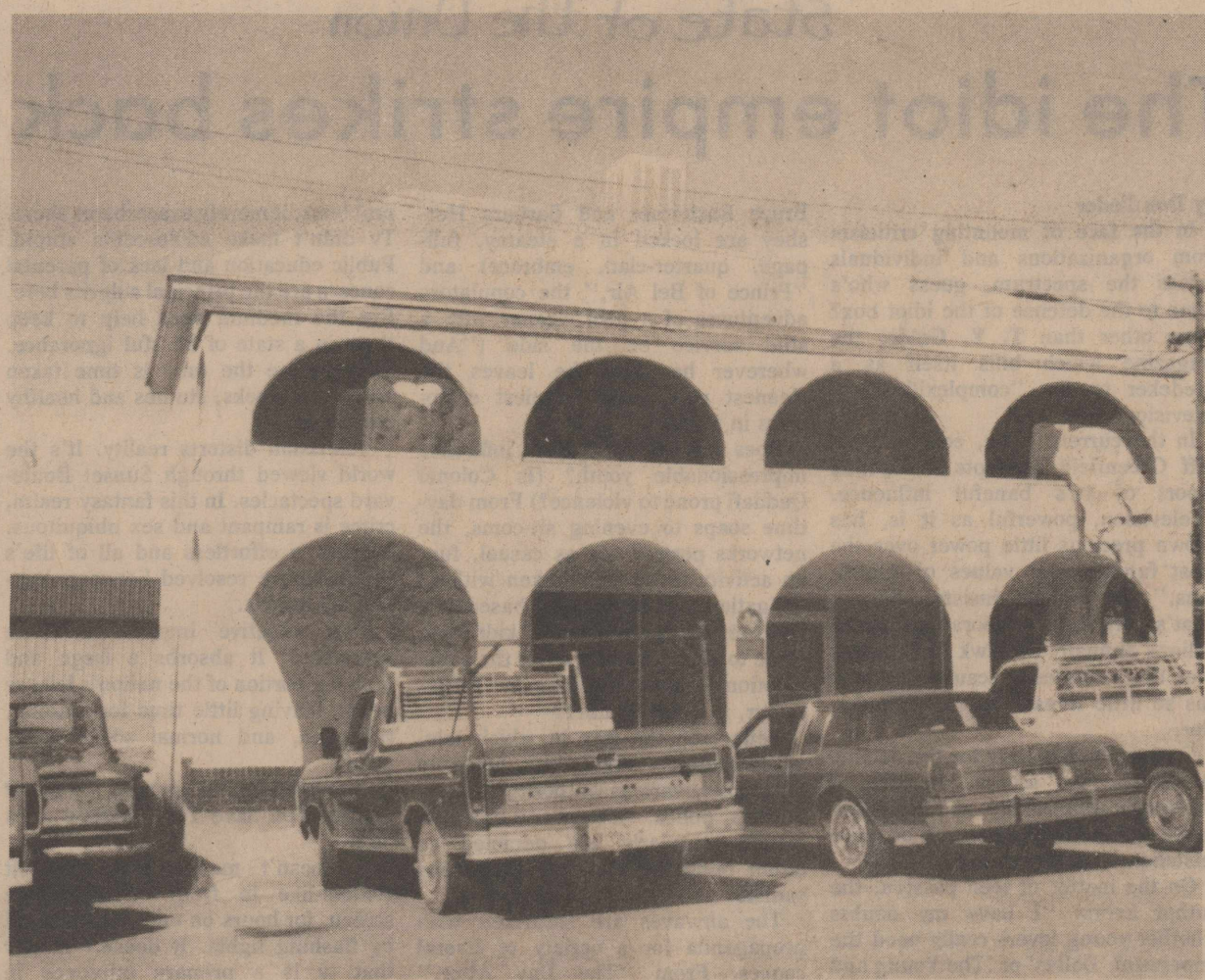
Eyesore in downtown Ozona The historical old Crockett Hotel has fallen into disrepair and broken windows are stuffed with old mattresses, a sad reflection on the historical marker which was placed there several years ago after restoration.
