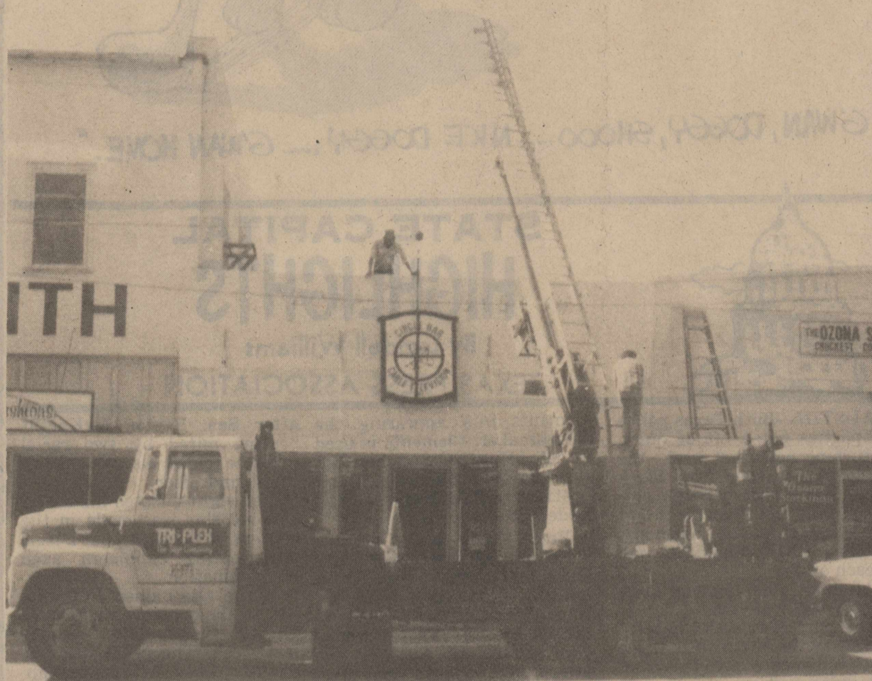
New lighted sign is installed
