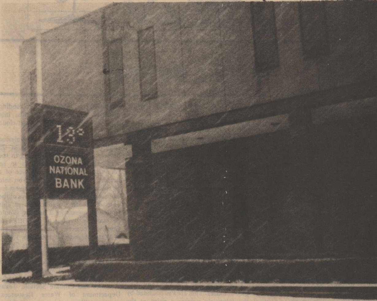
Height of the storm
