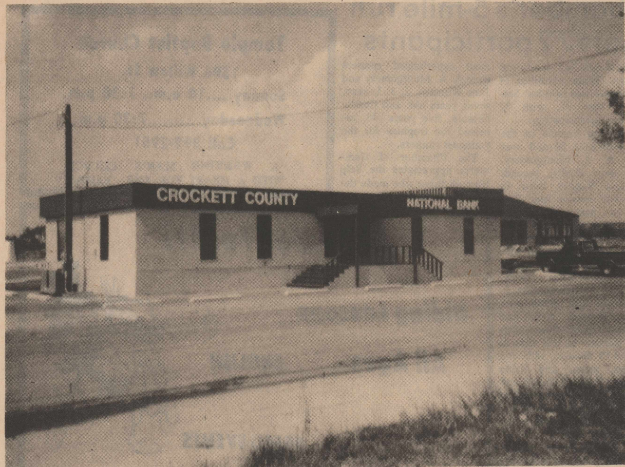
TEMPORARY QUARTERS for the new Crockett County National Bank will be open June 20. The building was moved onto the bank site and will be removed when the new building is finished early next year. Construction may be seen in the background.
