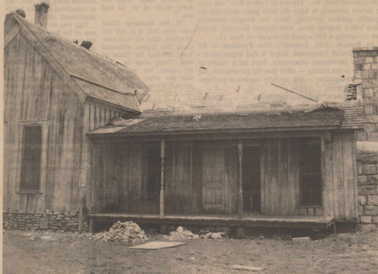
THE OLDEST HOUSE IN OZONA has reached its final resting place and is being restored at this site in Fairgrounds Park. The house will eventually be completely redone inside and out, and will be open for various
