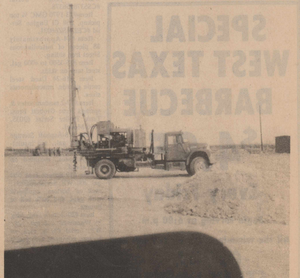
TWO MEN WERE INJURED here Sunday morning when this hole-digging rig became electrified with 69,000 volts of electricity. Sooner Williams and Douglas Ogelby had a narrow escape when the top of the rig they were operating came in contact with the major transmission line above. Both men suffered burns and were hospitalized.
