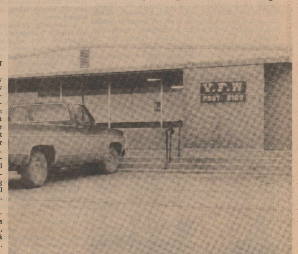
NEW HOME FOR VFW POST 6109 —Members of the Veterans of Foreign Wars have moved their post home to the old Montgomery Building which formerly housed the Trade Rite Grocery on Hwy. 290. The building is presently in the process of being remodeled, but is in use by post members.
