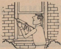
Caulk around doors and windows
