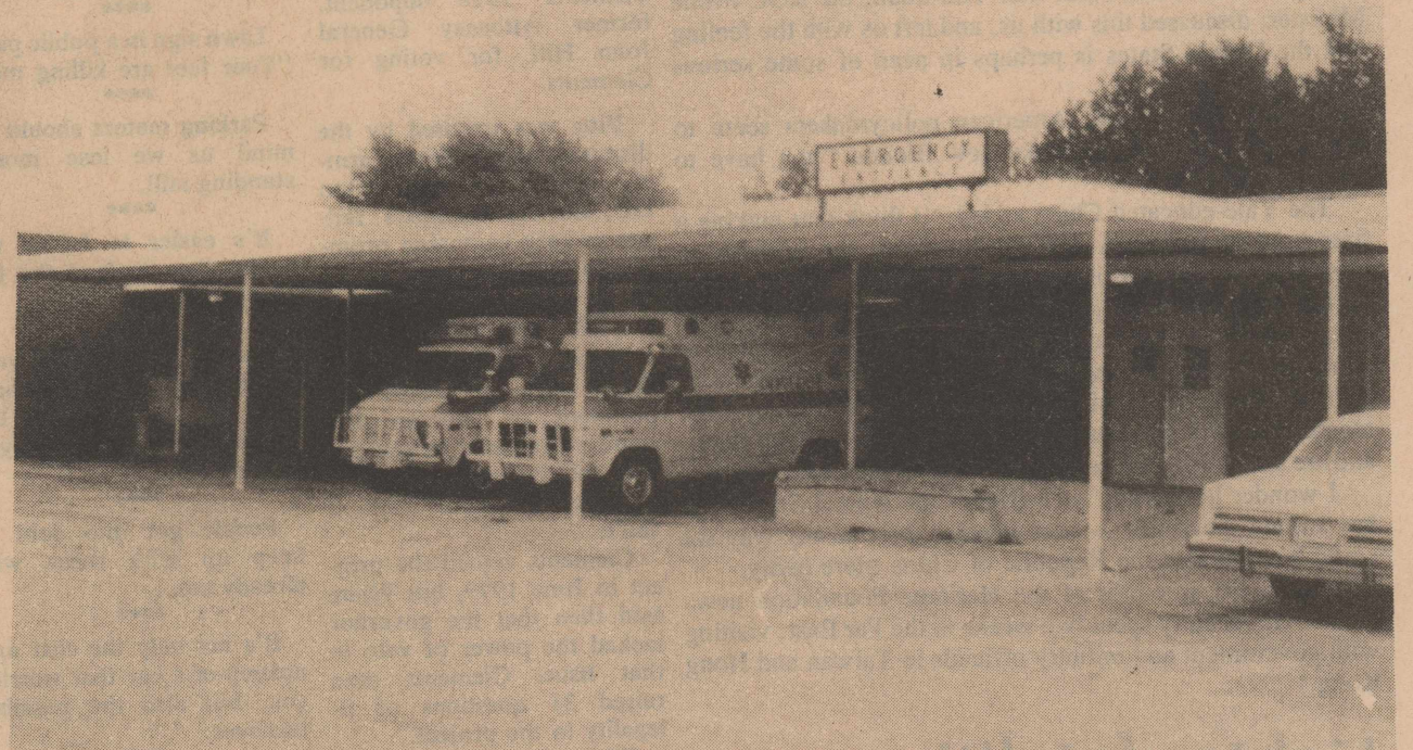
HOSPITAL IMPROVEMENTS recently completed include this covered canopy at the emergency entrance to the Crockett County Hospital, along with the lighted sign. The cover is designed to protect both ambulances when they are not in use for emergency service. A new policy initiated by
