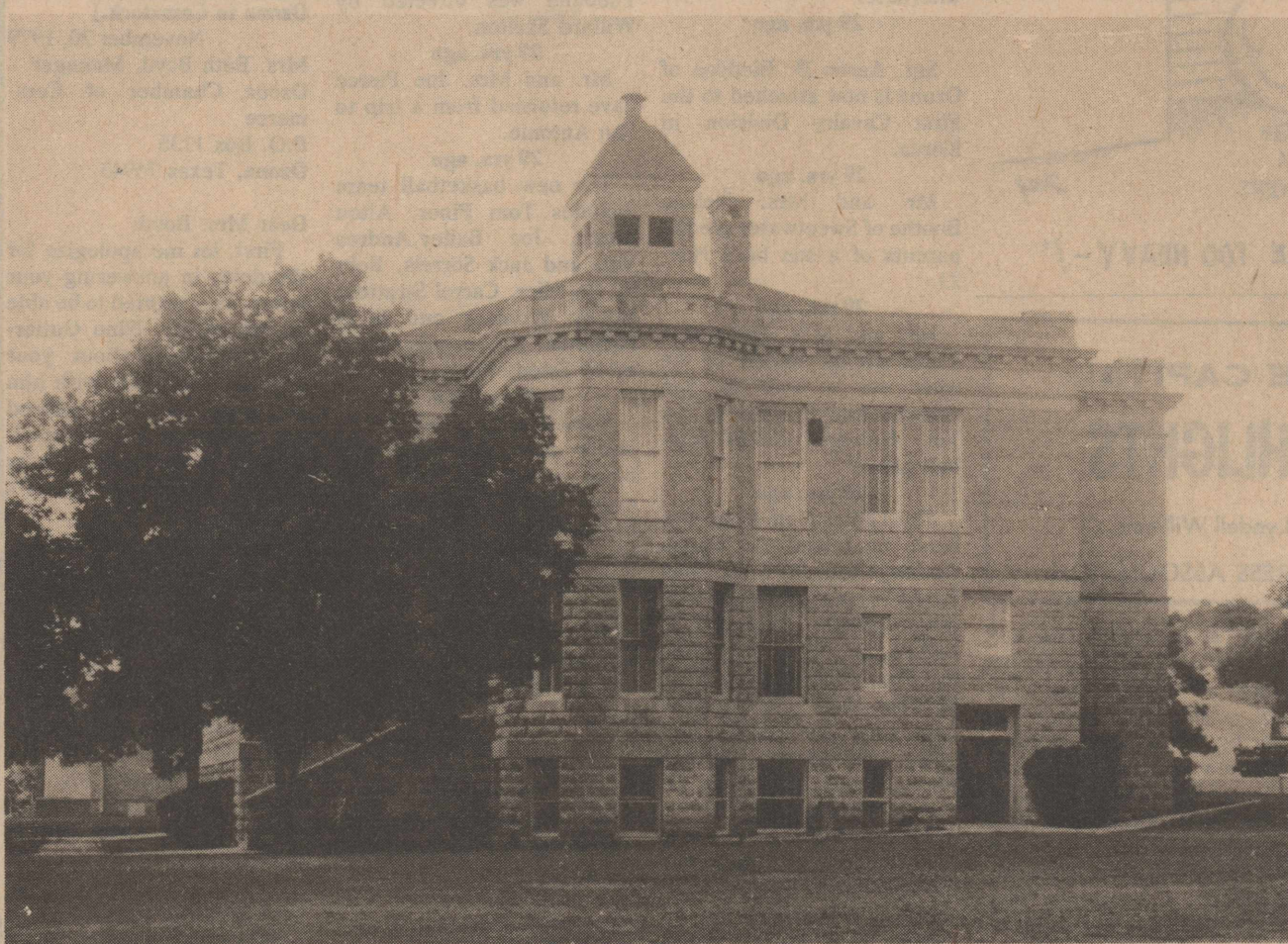
OZONA'S FIRST PERMANENT SCHOOL BUILDING built in 1912 and abandoned this year when the school improvement program moved the junior high students out of the building, was the subject of discussion Monday night at
