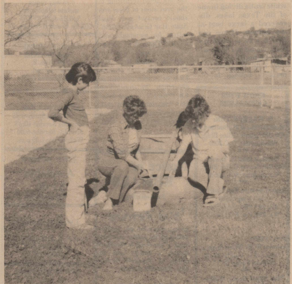
PLAYGROUND IMPROVEMENTS are in progress at the Ozona Community Center to accommodate a summer program for pre-school children. The fence has been erected by the county and here members of the Ozona Womens League, Judy Probst and Darolyn Webster, paint a basketball goal. Jennifer Probst looks on.
