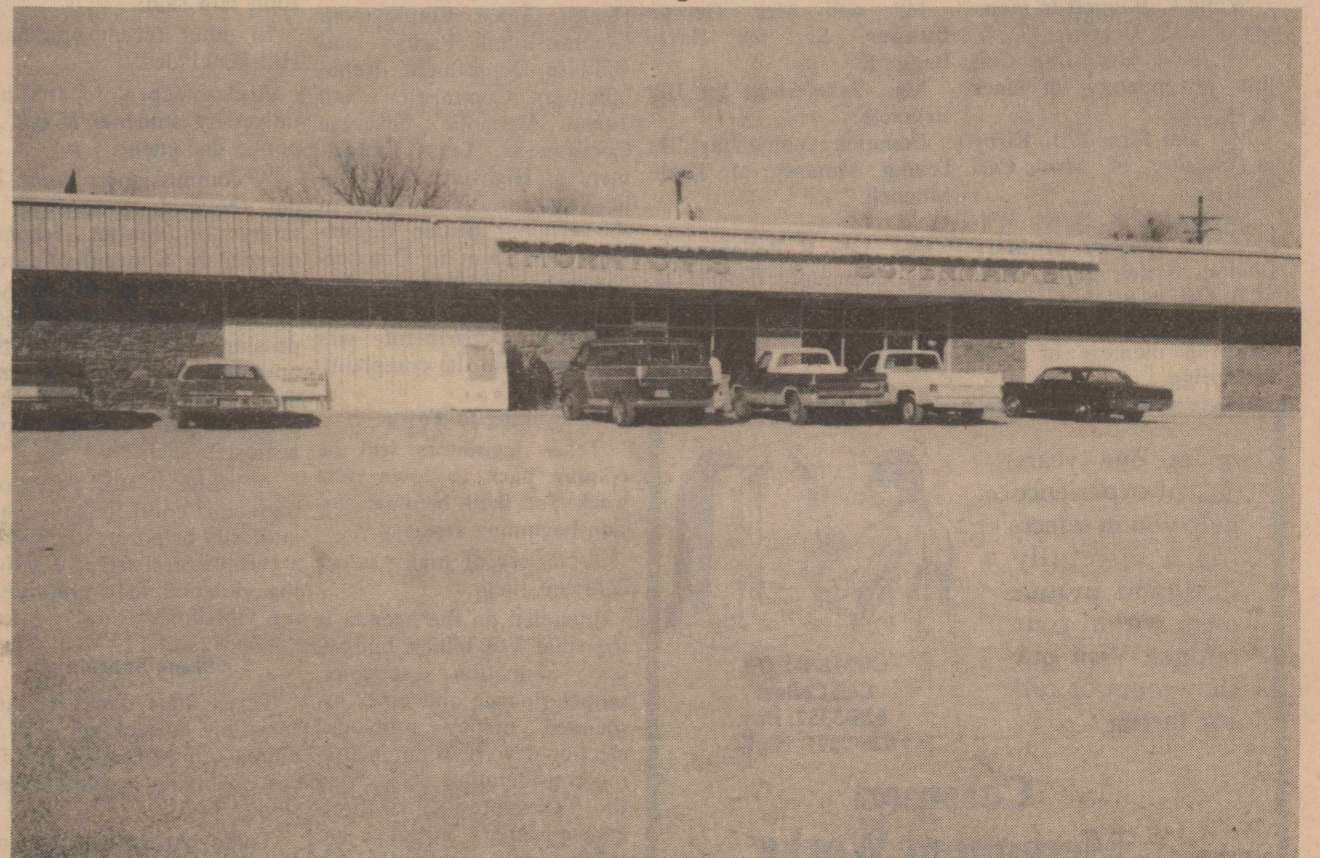
THORNTON'S SUPERMARKET OPENED AS SCHEDULED before the holiday rush. The spacious store offered a wide variety of fresh vegetables, fruits and holiday fare. The ample parking space assured customers of as much parking space as the new store offered shopping space.
