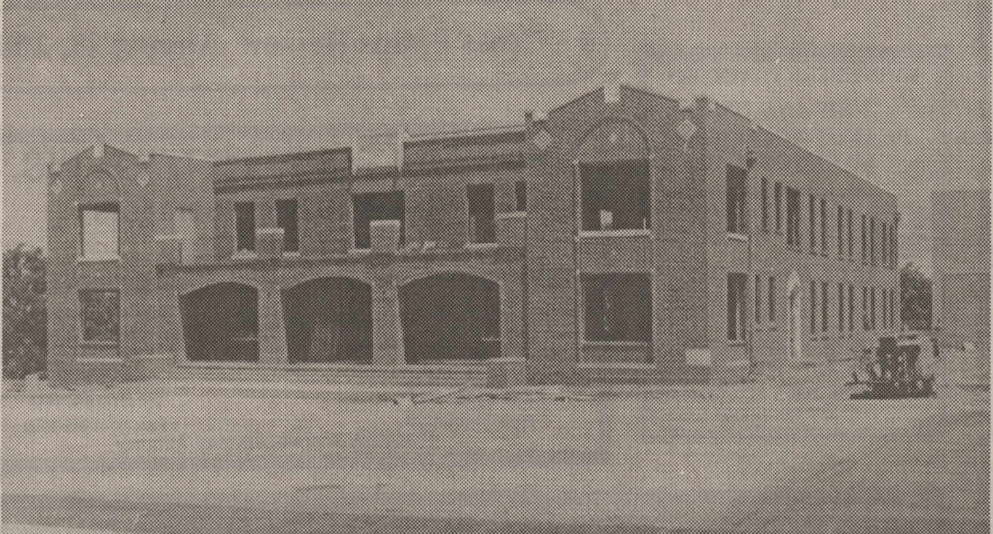
Renovations Underway At Bivins Hall At Cisco Junior College Campus
