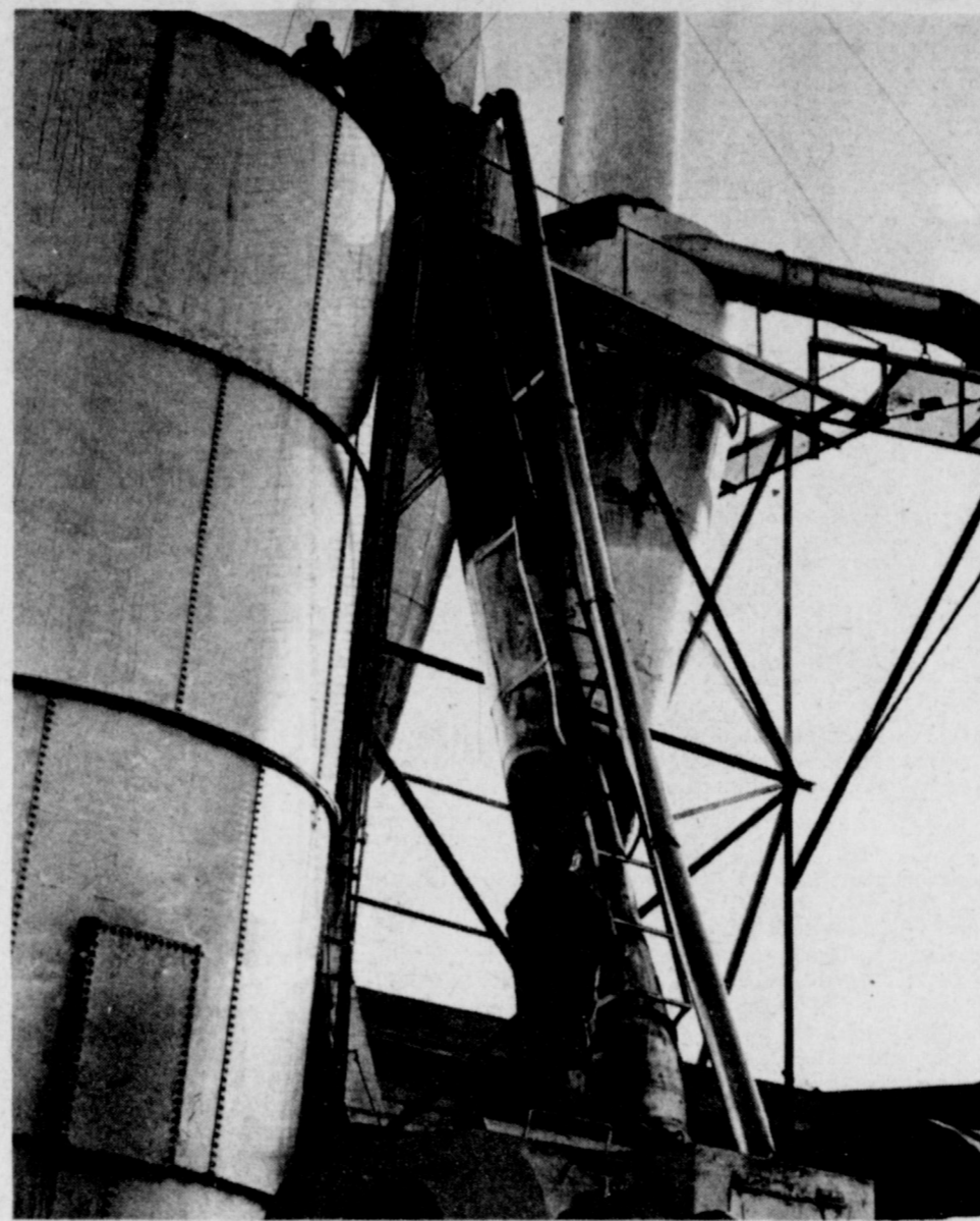
NATIONAL ALFALFA FIRE... A late Thursday afternoon fire did little damage at the National Alfalfa Dehydrating Plant in northeast Muleshoe. Pictured in silhouette are Muleshoe Volunteer Fire Department members who extinguished the auger blaze, which was apparently started from overheated alfalfa traveling in the auger.
