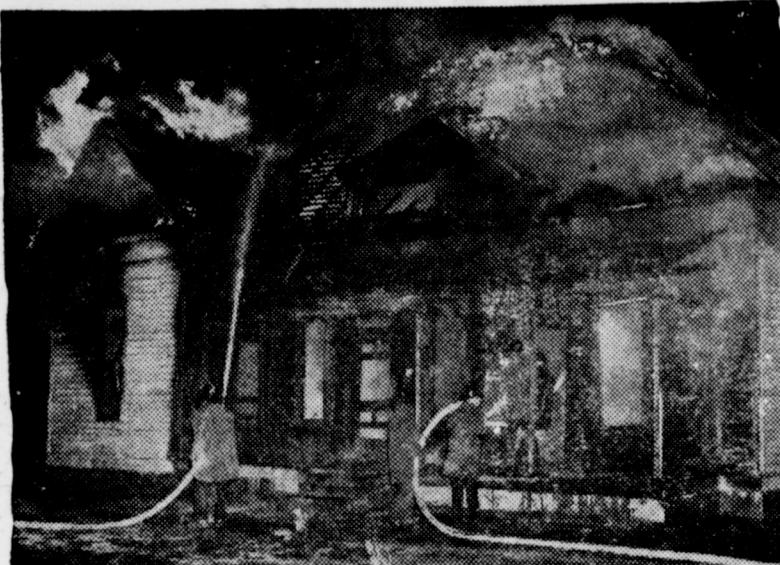
Flammable wood shingles enable fire to spread readily from building to building. In rural areas, whole farmsteads can be burned.
