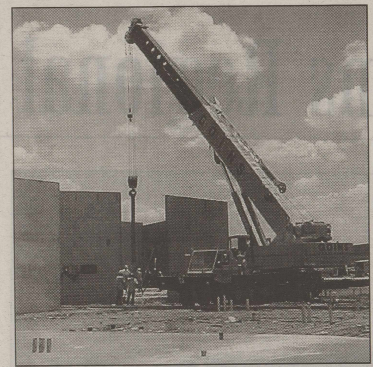
PRISON WALLS GOING UP —Heavy cranes tower above the skyline while lifting pre-formed cement slabs into place at the regional jail construction site.
