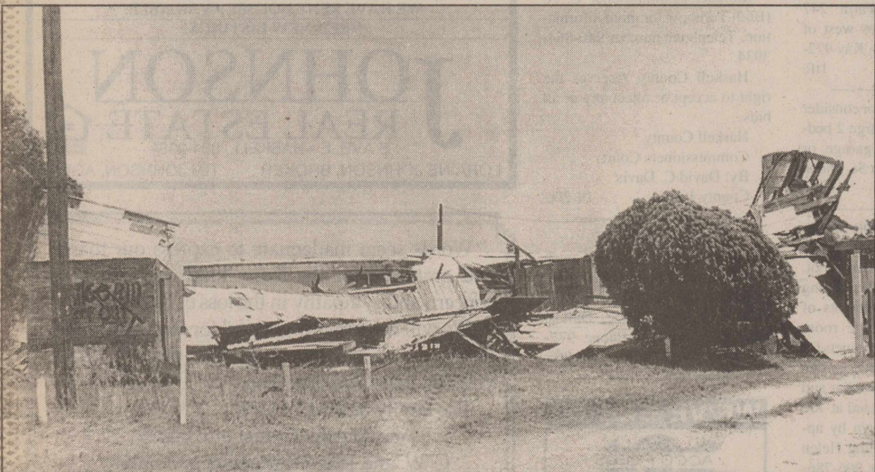
THEATER DAMAGE —Future plans for the historic Tower Theater of Rule were on hold following the wind damage last Fri. Allene Whorton, owner, said her hopes for a good season were sunk like the Titanic, which was billed to begin showing later that night. However, she said she hopes to reopen if possible. Saying that she began in the movie business in 1938, she added, "That makes me a veteran, I guess, and, like they say, the show must go on. Too many people depend on it for family entertainment."
