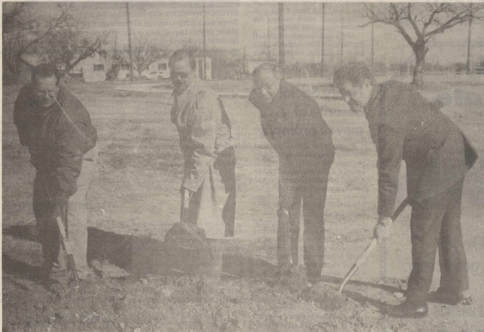
GROUNDBREAKING CEREMONIES —Groundbreaking ceremonies for the Kent Kwik Travel Center, located next to the City Park, were held last Thursday. On hand for the honors were from left,
