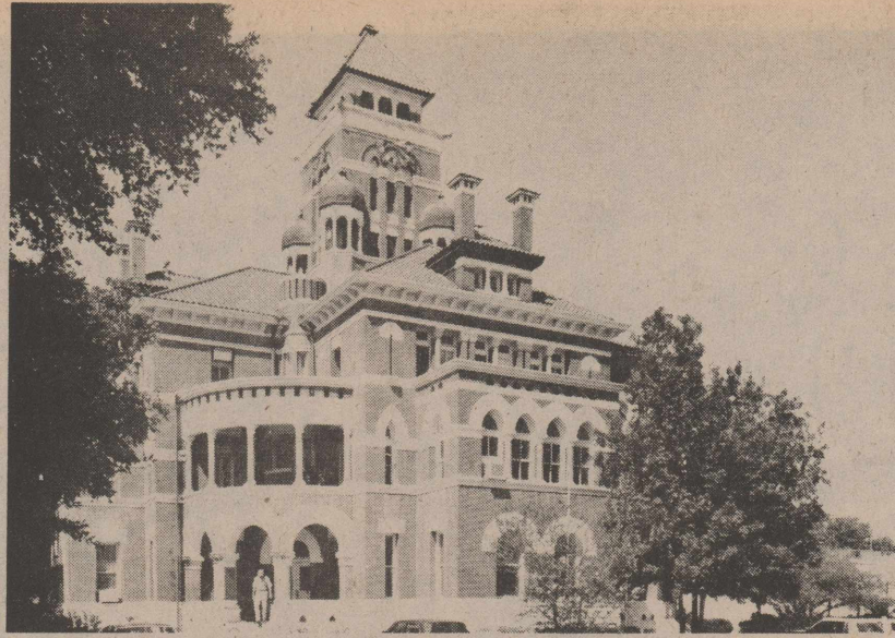
The Gonzales Courthouse in Gonzales County was completed in 1896 for a mere $64,450. It is the second such building for the 150 year old county, the first having burned in 1893. The town was once called the "Lexington of Texas" because the first skirmish of the Texas Revolution was fought here. Gonzales was named for Rafael Gonzales, the governor of the joint state of Coahuila-Texas in the 1820s. Today, Gonzales is a major producer of pecans, cattle and poultry. Tourism Division, Texas Department of Commerce photo.
