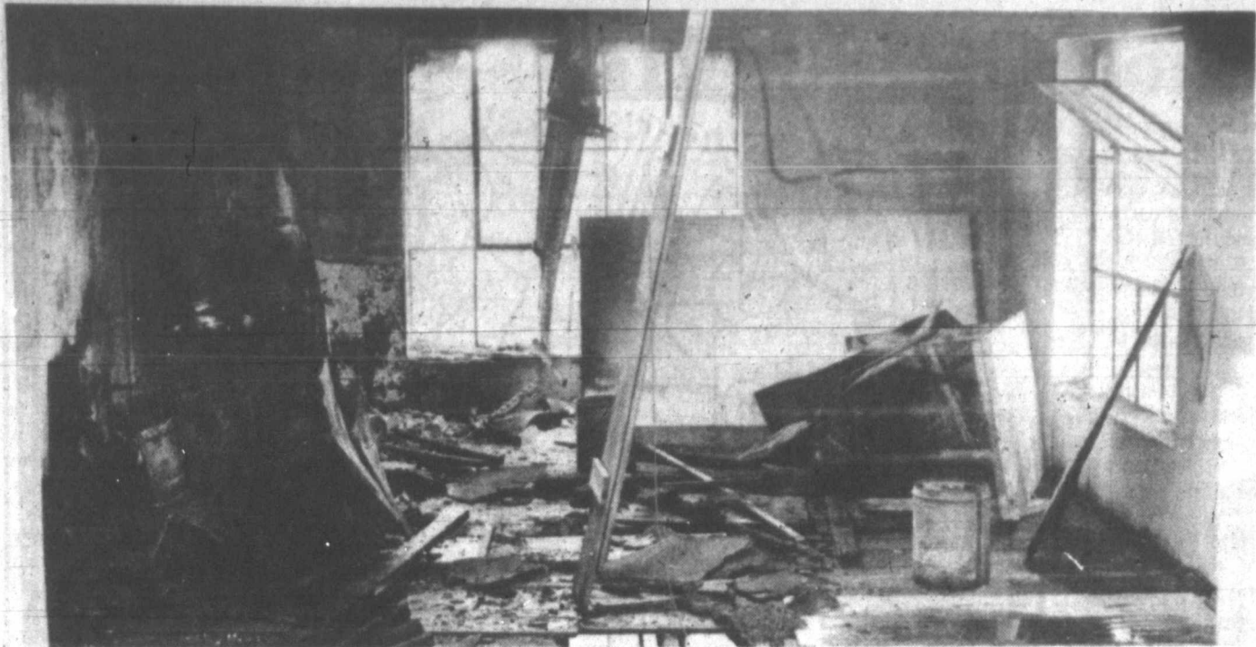
A TWO-STORY BUILDING in the 300 E. Francis block of Pampa received some heavy damage Monday following a fire. Pampa firemen were called to the scene at 2:10 p.m. and the blaze was put out less than 10 minutes later. Fire Captain Don Hendricks said heavy damage was done to the upstairs southwest corner, which is shown above. Fires had been started at the building two or three times in the past year. The building, which has been vacant for seven
