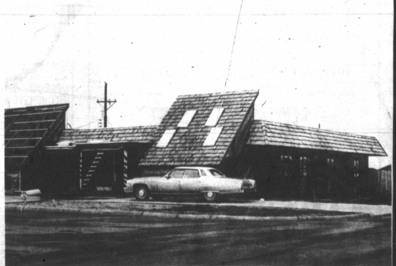
A full view of the first house in Pampa equipped for solar heating. The picture shows four of the 13 skylights.
