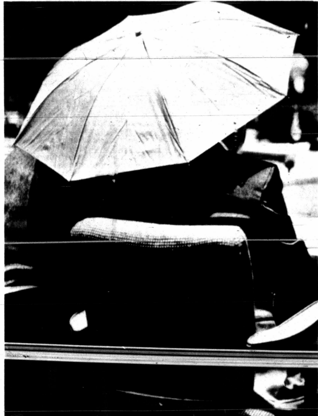
REPS. LARRY BAHILL, D-Tucson, and Larry Hawkes, R-Tucson, use an umbrella to protect them after the roof sprang a leak in the Arizona House of Representatives chamber Wednesday. The leak didn't interrupt regular House business. (AP Laserphoto)
