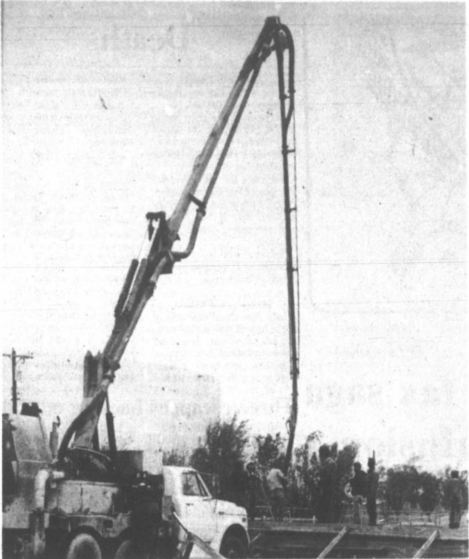
**PAMPA CONCRETE** using a special pump truck to pour concrete at the new 4-R Supply location. The special truck is only used on jobs that regular trucks can not reach.
