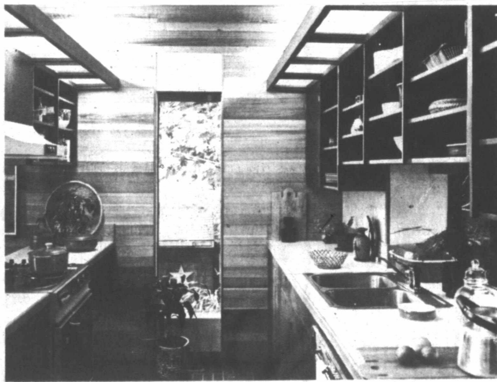
Pullman or corridor-type kitchen, with open upper shelves of 1 x 12-inch western wood boards, organizes meal preparation, saves unnecessary steps. Fluorescent tubes above frosted glass set in frames of fir 2 x 4's and 1 x 4's provide soft, indirect lighting for the working areas.
