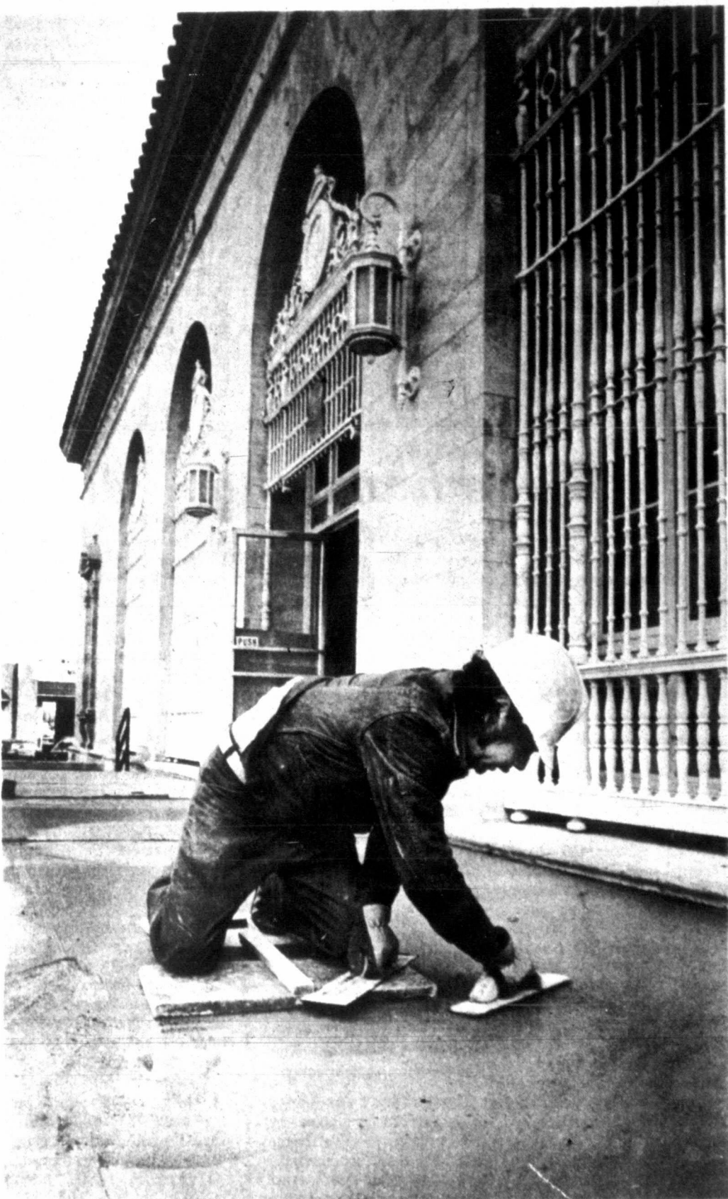
Concrete laid at post office
