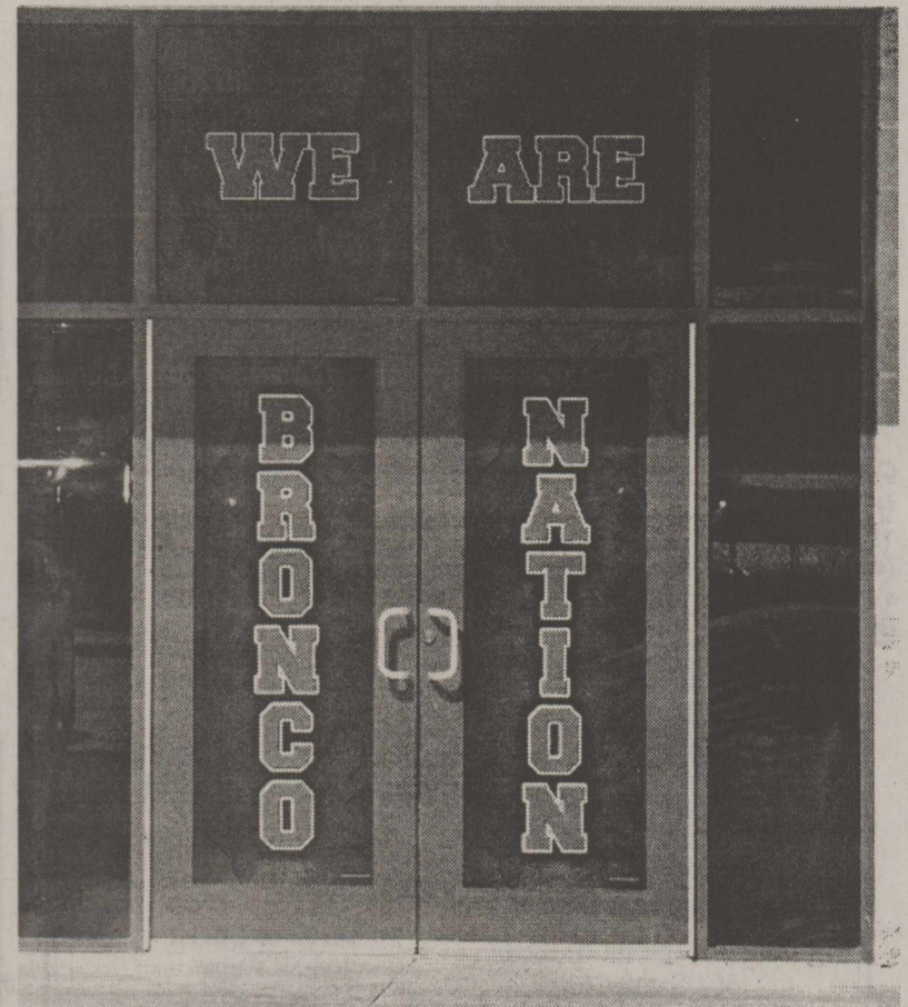
The refurbished Bronco Field House has a new entrance.
