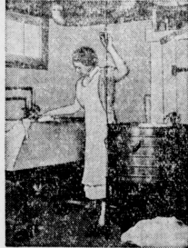
Washing machines must necessarily be used in the vicinity of water so that electric connections are advisable. Convenience outlets with insulating covers preferred to pendant cords. Metal sockets as shown here should not be used in this location.
