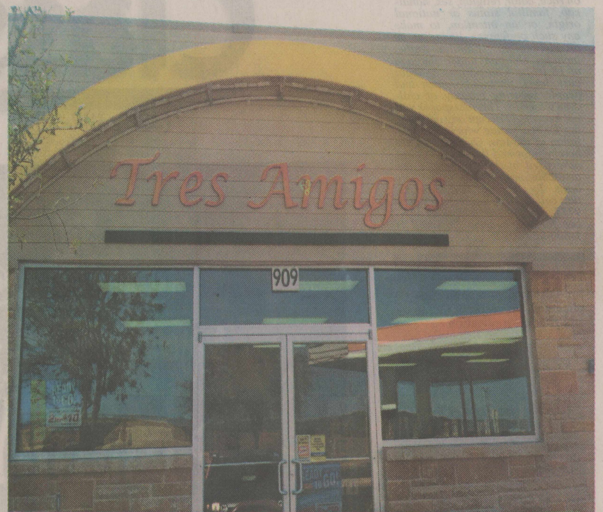
The remodeling is finished on Tres Amigos Convenience Store located at 909 Water Street. The hours of operation 6:00 a.m. to 11:00 p.m. 7 days a week.
