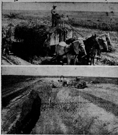
TRENCH SILOS POPULAR IN BAILEY COUNTY
