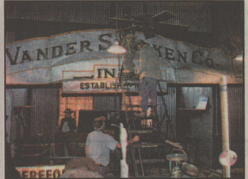
David Walsh crew installing the Vander Stucken sign in the Ranch Museum.
