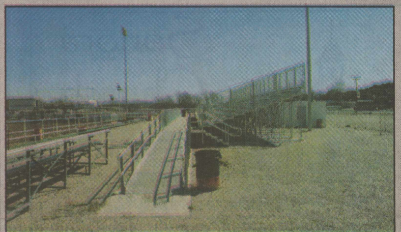
The grandstands at the Sutton County Arena stand bare, awaiting the construction of a new cover as well as many other improvements.
