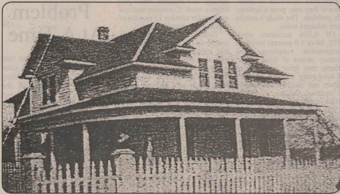
Original Lowrey House before the up-stairs and porch were removed.
