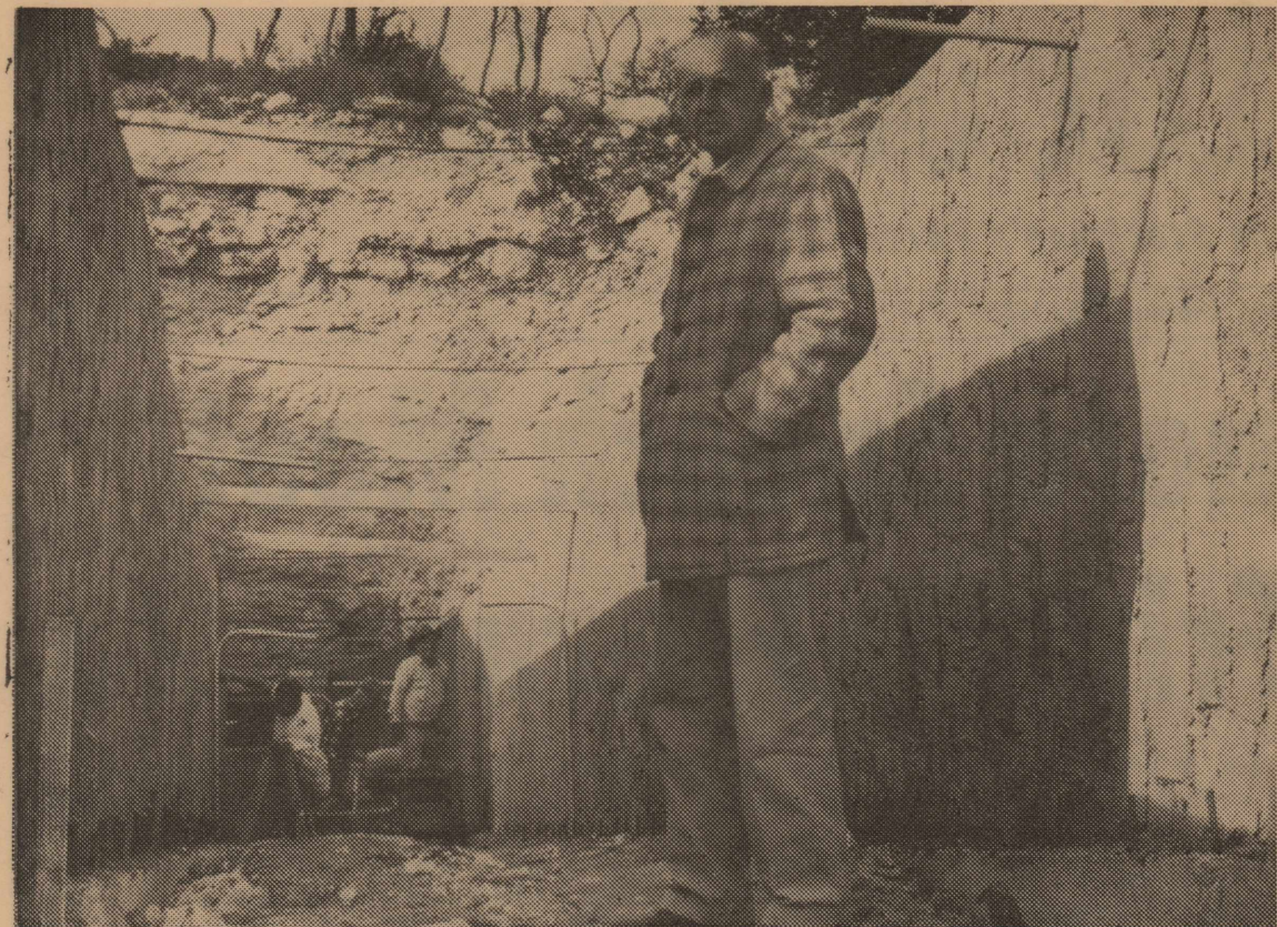
JAMES MORKKIS , manager of the Sonora Caverns, supervises work on the tunnel being built at the exit of the cave. The tunnel will enable tourists to leave the cave by gradually ascending up a ramp to the surface rather than climbing many flights of stairs upward.
