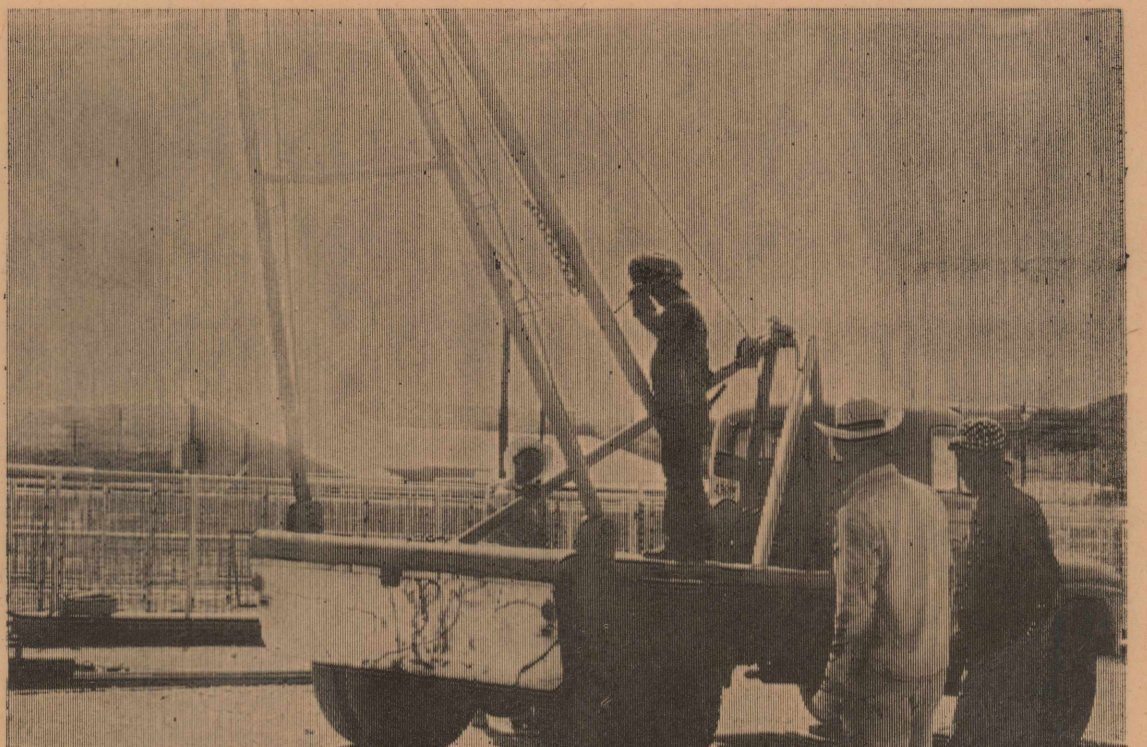
City workmen stand by while electric wench is being moved into place at the Sonora Stockyards.
