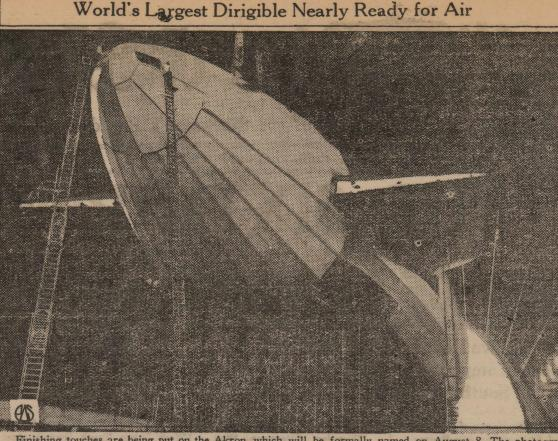
Finishing touches are being put on the Akron, which will be formally named on August 8. The photograph shows the three fins in place and the outer covering being applied to the ship's tail. Each fin is forty feet wide and 105 feet in length. The Akron is 785 feet long and weighs 221,000 pounds. It can lift 182,000 pounds of "pay load" besides its own weight. Mrs. Hoover will christen the airship by liberating a flock of doves.
