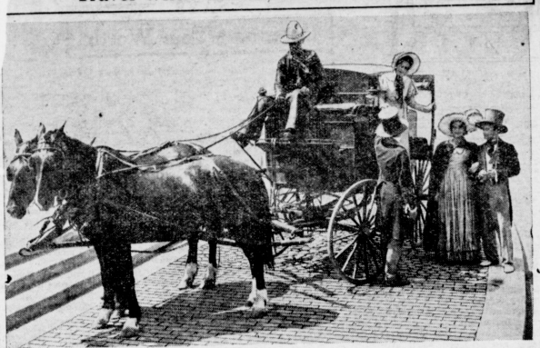
This is a scene typical of Dallas and its Main Street of early days. The photograph was taken on one of the nine famous roads and highways which have been reproduced by the Ford Motor Company at the Texas Centennial Exposition in Dallas. In 1851 the street was paved with round bois d'arc blocks and later on the round block was replaced with rectangular blocks. Both types are pictured here.
