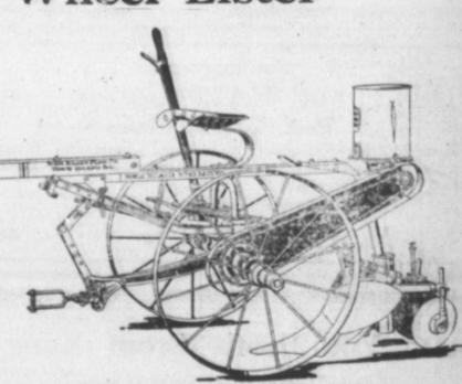
You not only have an accurate dropping system on this lister for either cotton and corn, but you also have the big advantage of being able to see at all times that it is planting accurately. The seed spout and delivery are at the front of the hopper instead of the rear. It is a very simple matter to glance to the rear, see just how your lister is planting and make certain that the hopper is not empty-without stopping your work.
