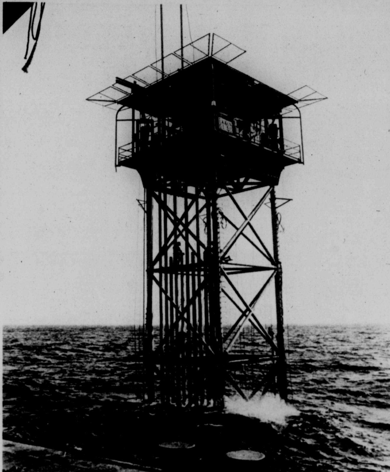
NEW-TYPE OFFSHORE drilling and production platform designed for use in deep waters is installed offshore Louisiana for testing. The experimental tower is held in vertical position by underwater guy lines attached to anchors. If successful, the experimental structure designed and
