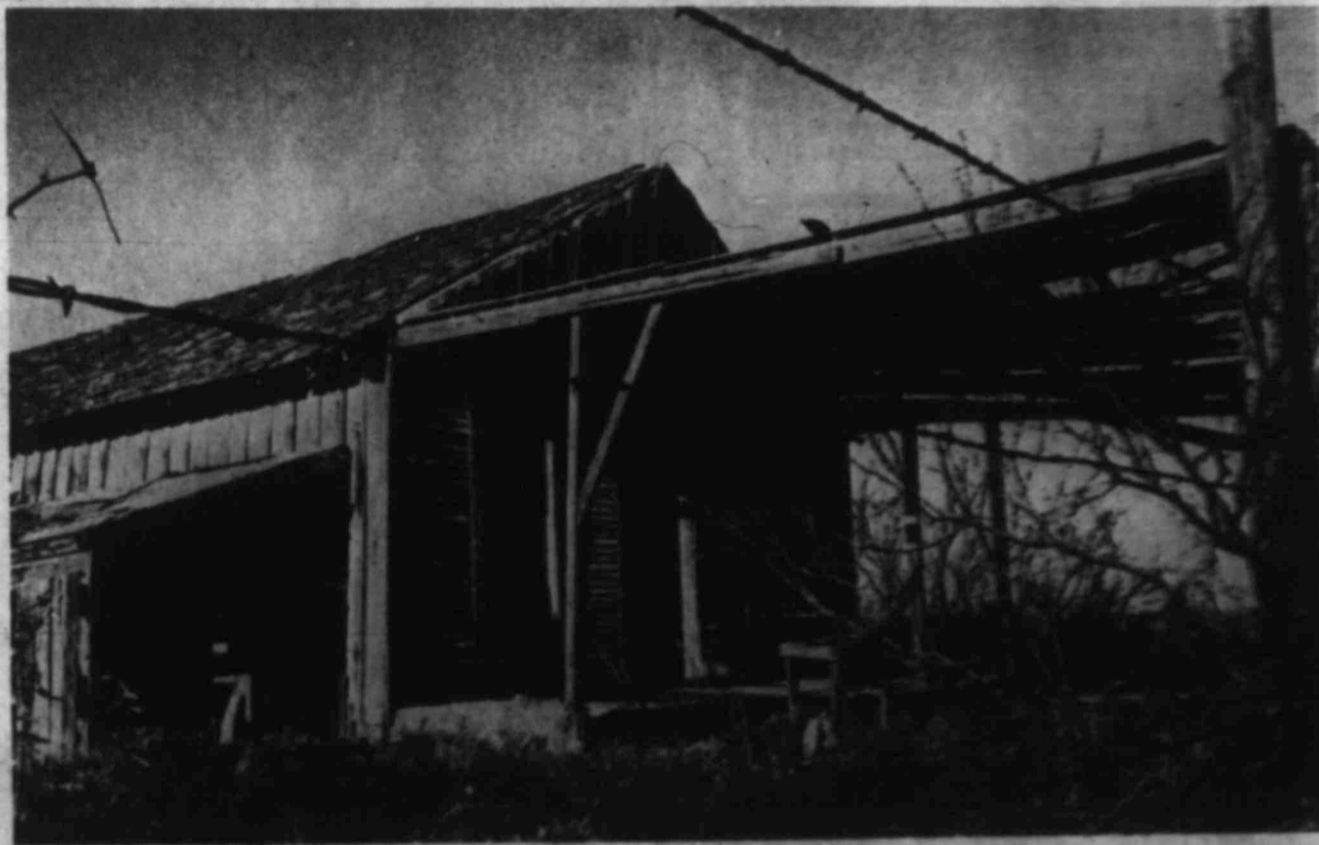
TIME AND WEATHER have taken their toll on this old building east of Midland. It was once the center of the community of Germana. The story of Germana and other pictures of the way it looks today are on Page 10A.
