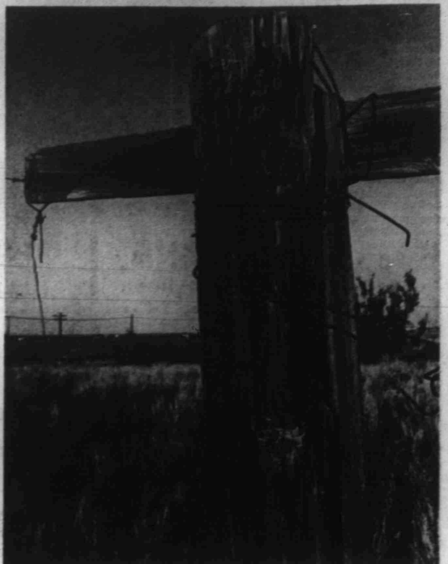
A length of wire wrapped remains of a once-useful clothesline in Germania.
