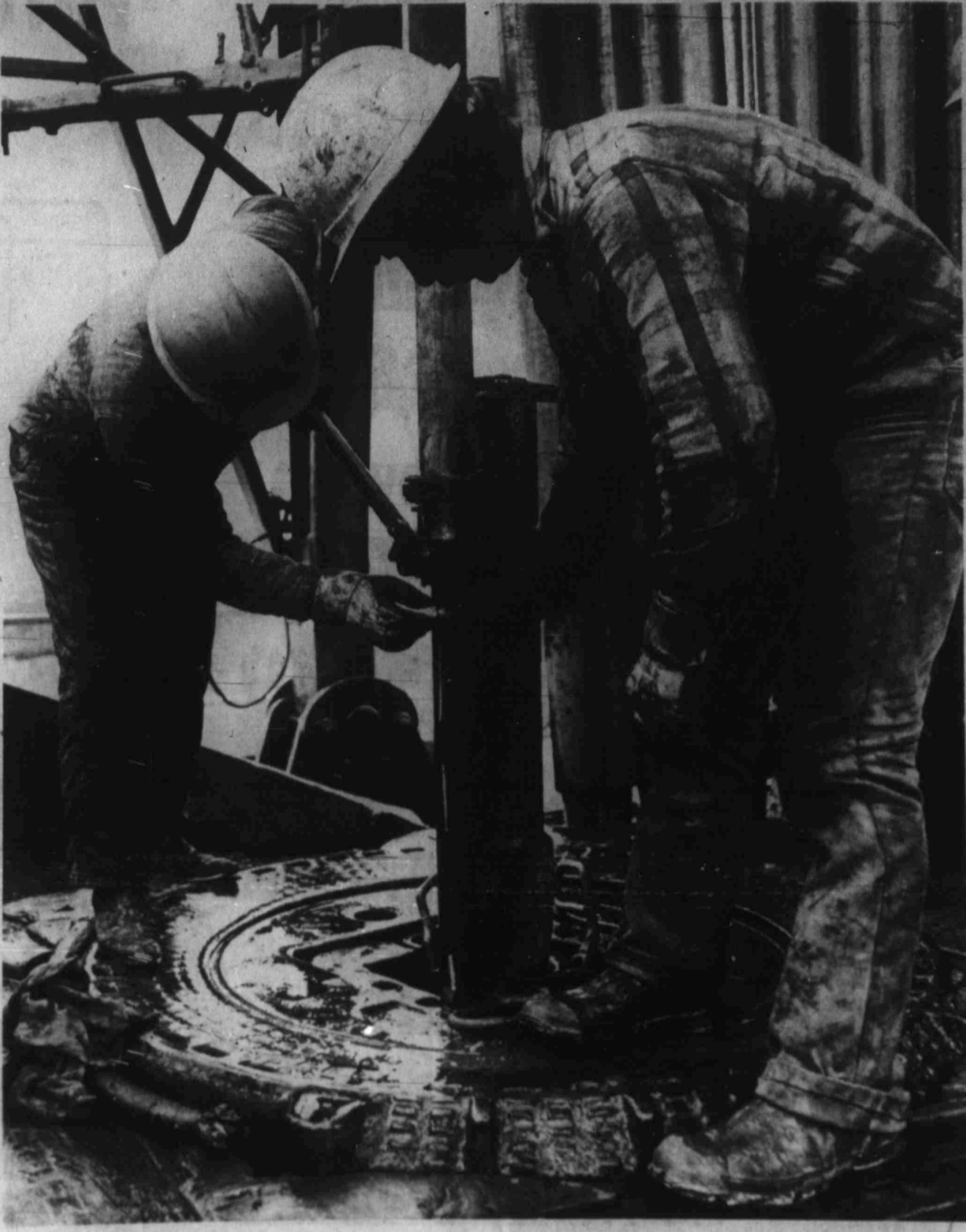
WORKERS MEASURE A rock core as it is extracted from a well located in Gratiot County, Mich. Scientists hope the core will help to determine where Michigan lay millions of years ago in relation to the ancient North Pole.
