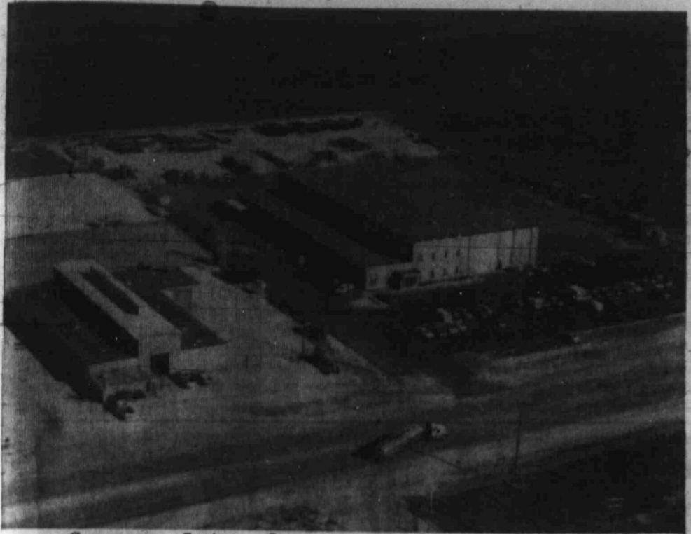
Compressor Systems, Inc., completed the two-story addition at right to its complex at Terminal during October.
