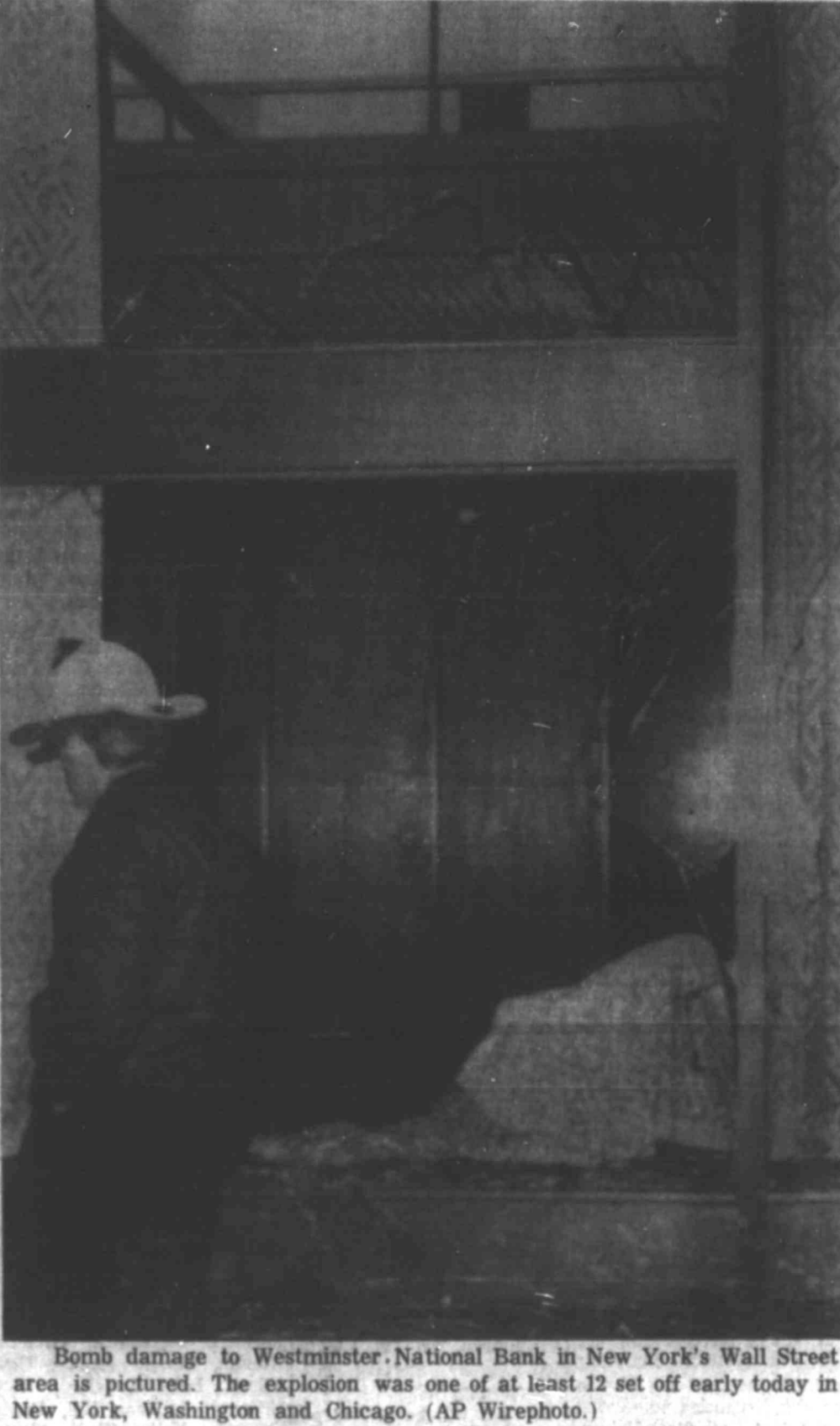
Bomb damage to Westminster National Bank in New York's Wall Street area is pictured. The explosion was one of at least 12 set off early today in New York, Washington and Chicago. (AP Wirephoto.)
